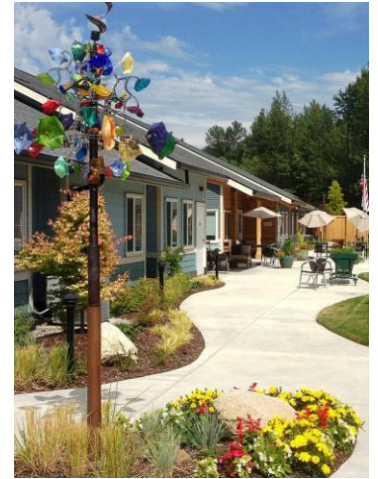
Edgewood Special Care Community; Edgewood, WA
