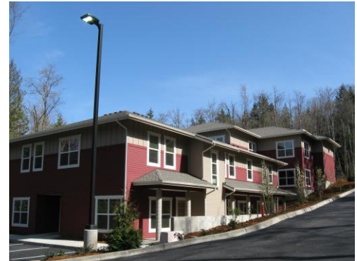
Keller House; Bremerton, WA
