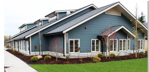
Edgewood Special Care Community; Edgewood, WA
