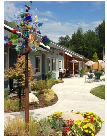
Edgewood Special Care Community; Edgewood, WA
