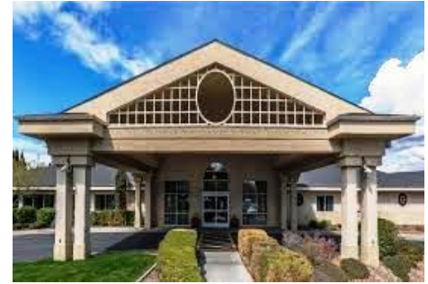
Regency Wenatchee Rehabilitation and Nursing Center; Wenatchee, WA
