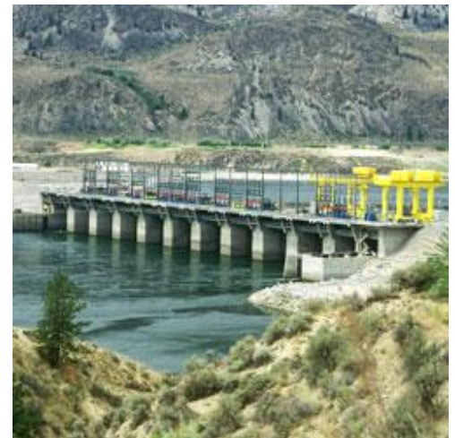
Wells Dam; Chelan County, WA
