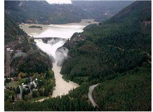
Newhalem/Diablo Hydroelectric; Newhalem, WA
