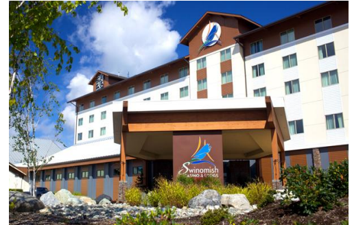
Swinomish Hotel and Casino Expansion; Anacortes, WA
