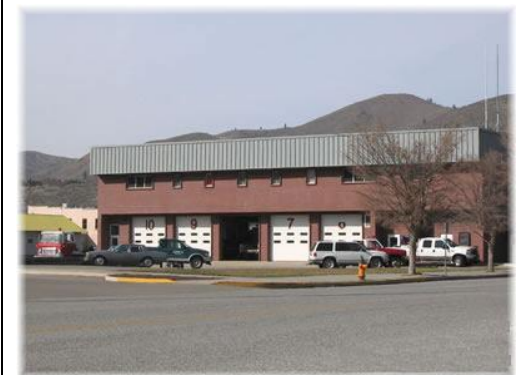
Chelan Fire Station; Chelan, WA
