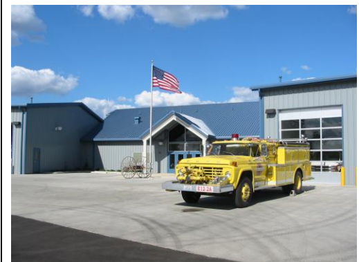
Lewis County Fire Station #12; Centralia, WA
