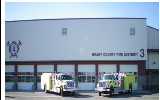
Grant County Fire Station #3; Quincy, WA
