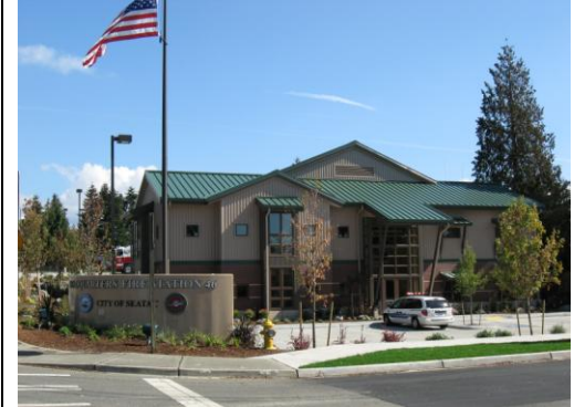
SeaTac Fire Station #46; SeaTac, WA
