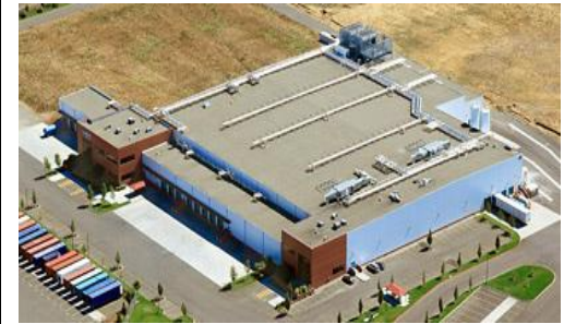
Millard Cold Storage; Centralia, WA
